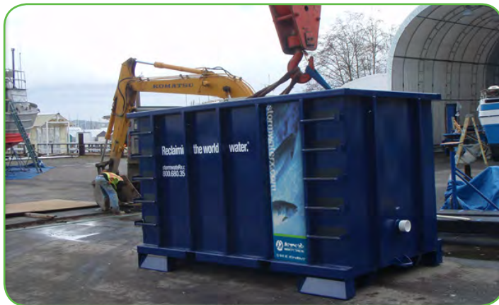
Installation of an AquiP 50 system
